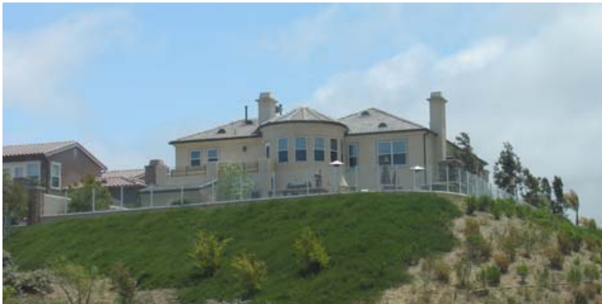
Figure 38 Urban use of recycled water in the IRWD
