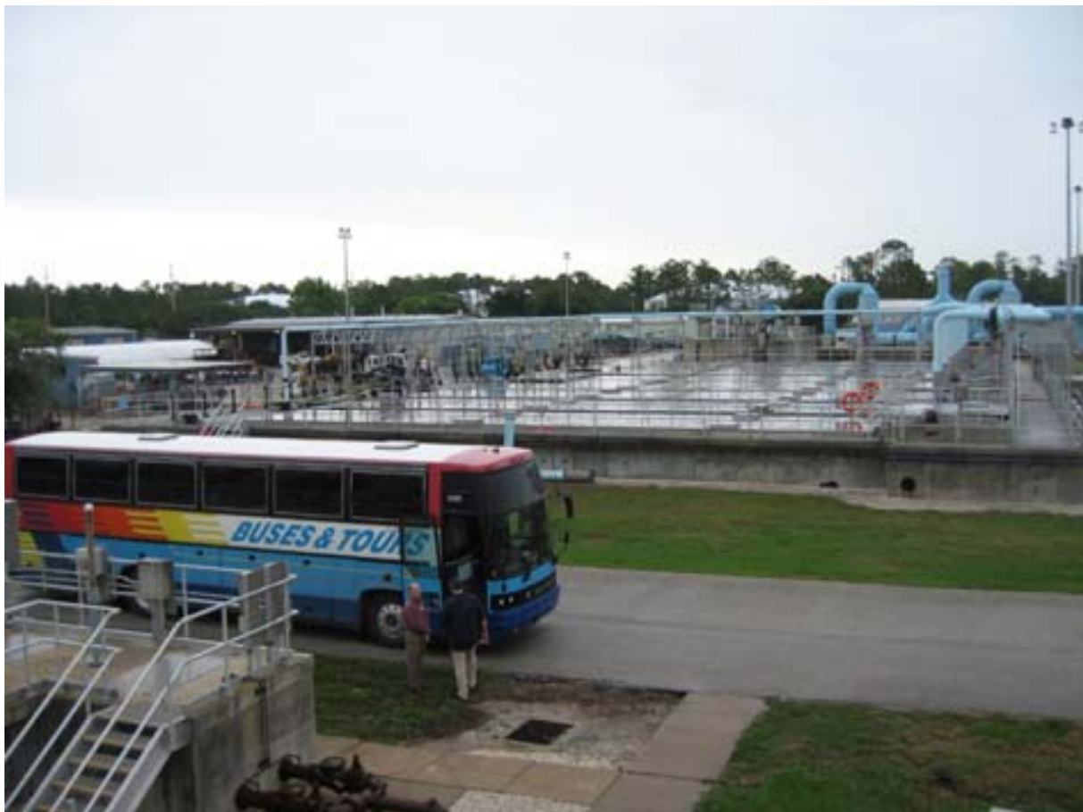
Figure 12 Wastewater Reclamation Facility at Reedy Creek/Disney World, Florida.
