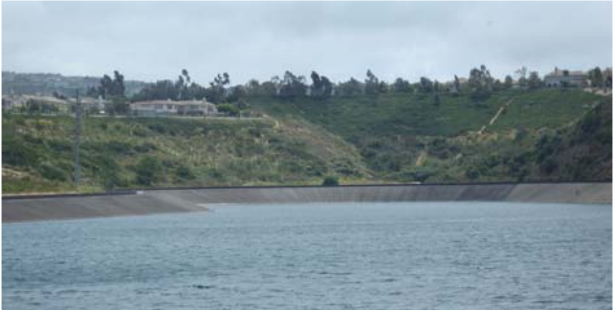
Figure 39 Old potable water reservoir used for storing recycled water, IRWD, California.
