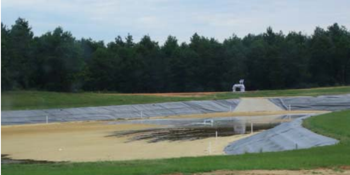
Figure 4 Rapid Infiltration Bay (RIB) where recycled water is stored and can move into the soil and eventually the aquifer at a rate of up to 30 inches per day.
