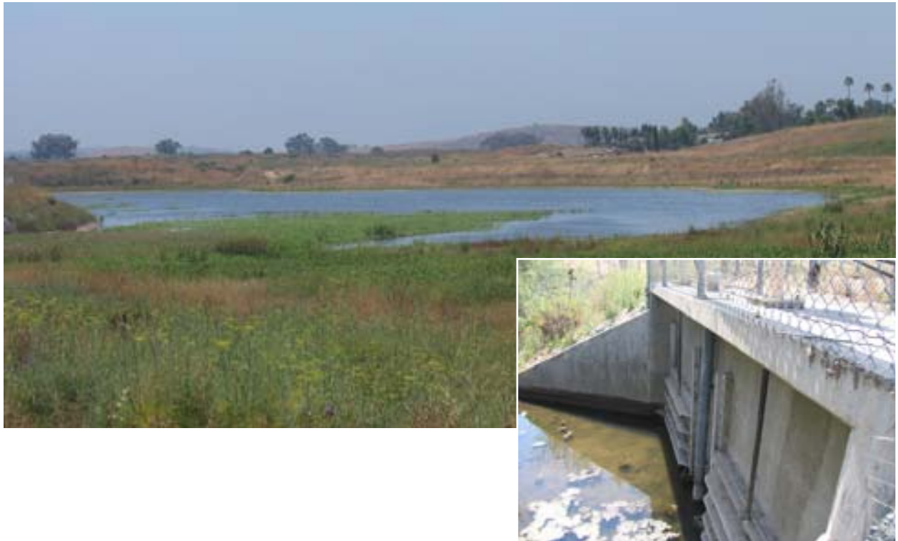
Figure 30 Urban Runoff Diversion System lake and first flush diversion gates.
