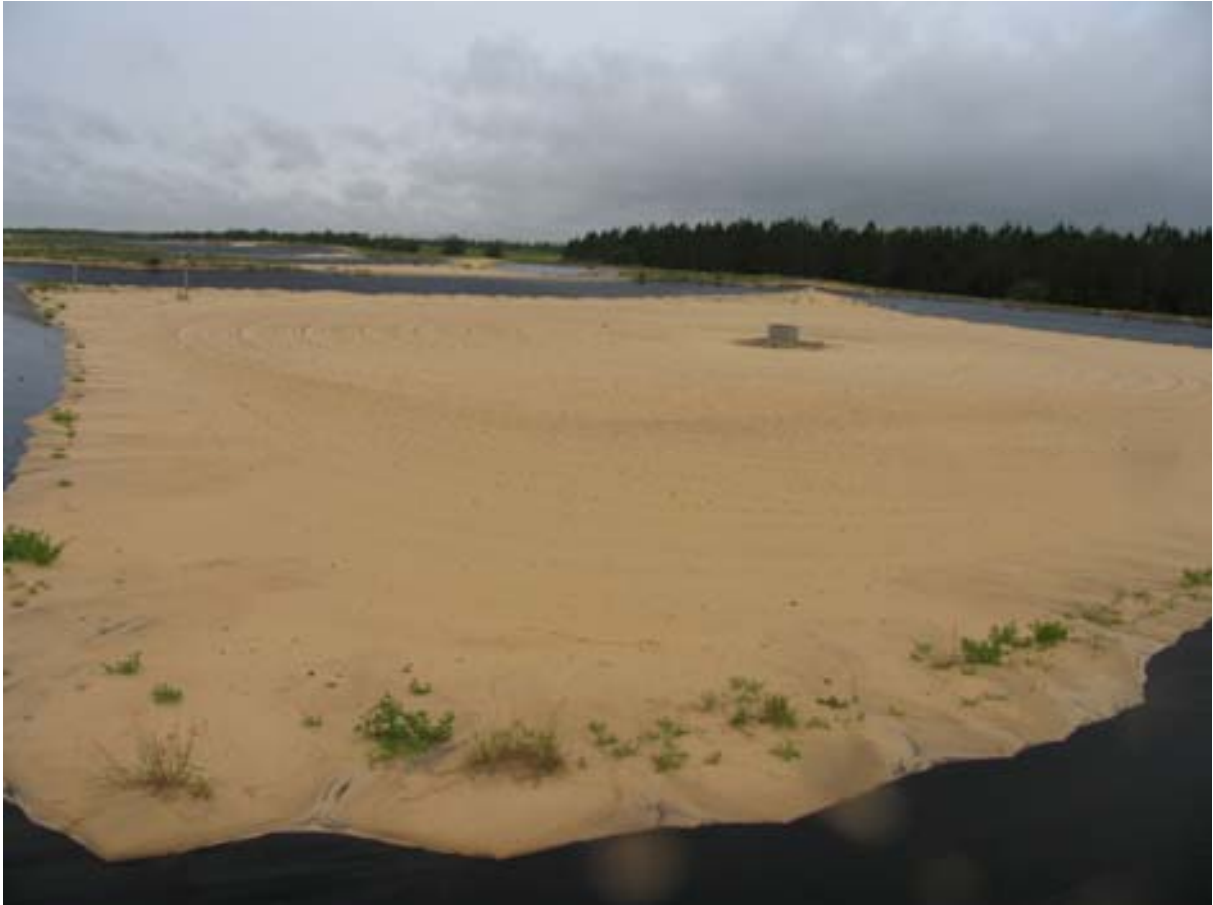
Figure 14 Rapid Infiltration Basin (RIB) – Reedy Creek Energy Services. Disney World, Florida.
