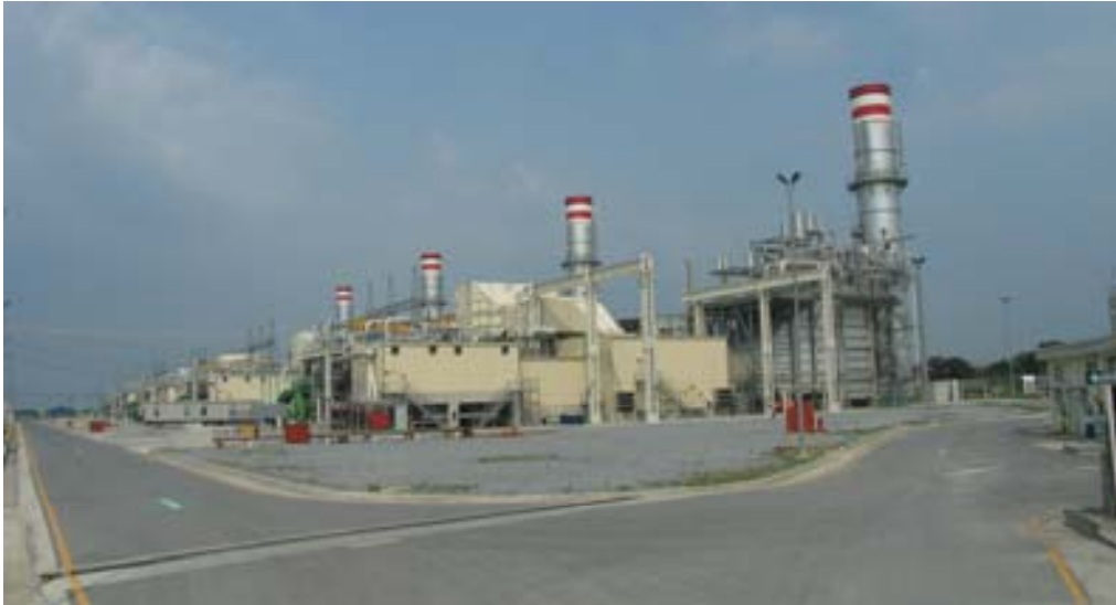
Figure 26 Power generation plant at Iberdrola, N.L. Mexico.
