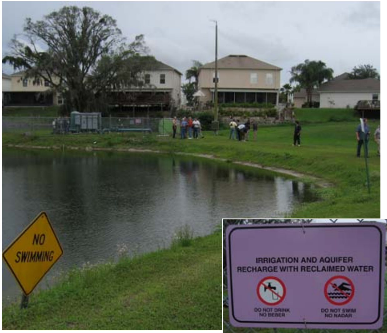
Figure 10 Recycled water storage dam backing on to residential housing and signage used (insert), City of Sanford, Sanford, Florida.
