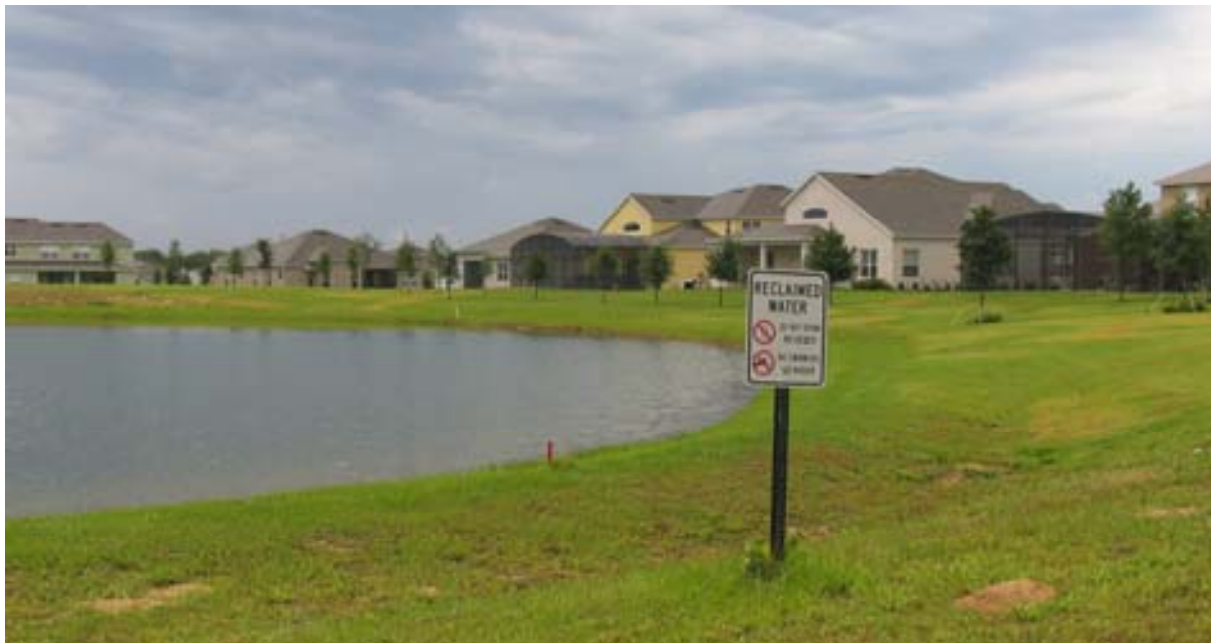
Figure 8 Reclaimed water storage pond within the residential development at Rock Spring Ridge Residential and Golf Development, showing some of the signage. We weren't too sure about the risk from golf balls to children playing in the playground?
