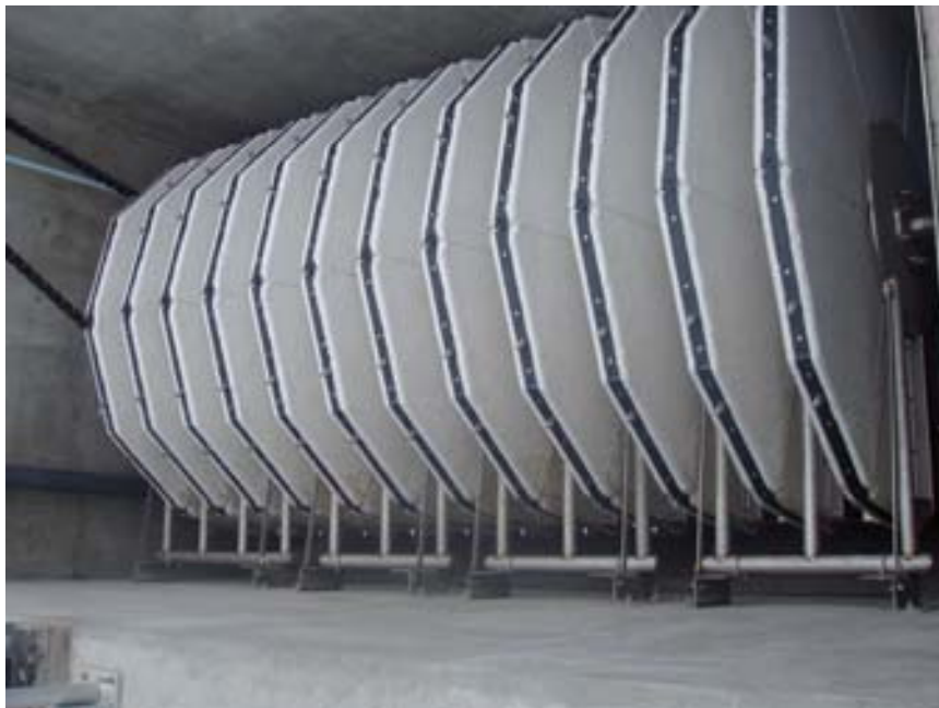
Figure 21 Cloth disk filters at the North WRF, Manatee County.
