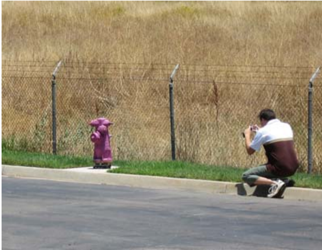
Figure 32 Reclaimed water fire hydrant at the Padre Dam Municipal Water District Wastewater Treatment Plant.
